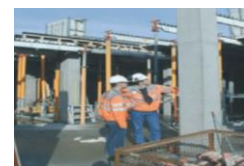
Green concrete column
